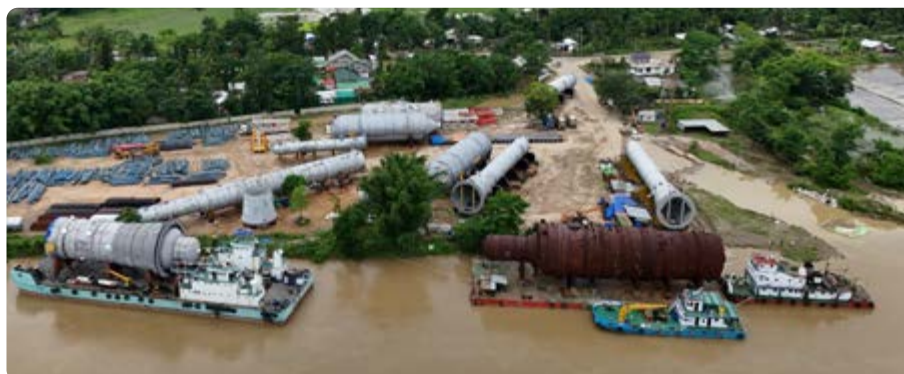
Jetty in Dhansiri River to receive ODC through water ways
