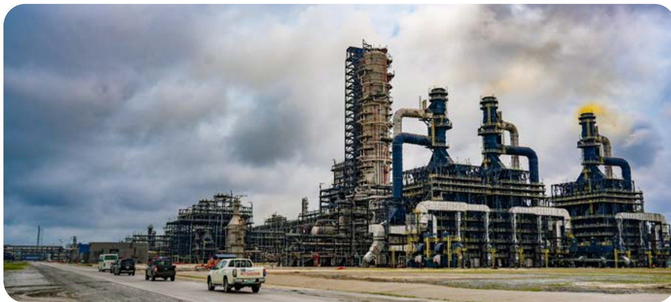
Dangote Refinery Project, Nigeria
