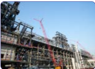
Installation of Demo Bio ATF unit of MRPL
