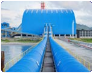
Direct Reduced Iron (DRI) plant
