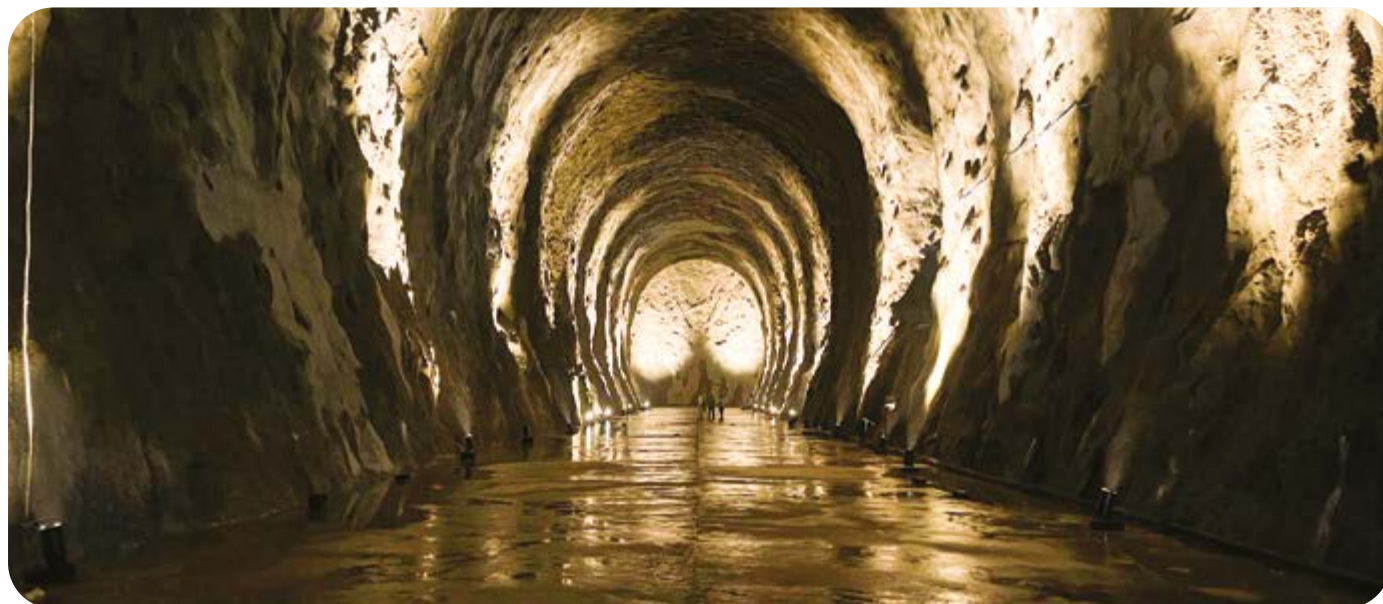
LPG Cavern Project in Mangalore
