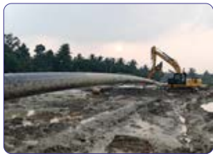
Dobhi-Durgapur-Haldia Pipeline Project
