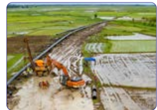
Upgradation of facilities for Numaligarh-Siliguri Pipeline
