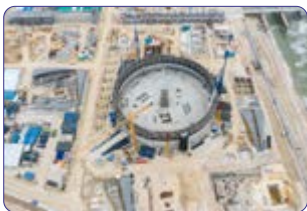
NHT-CCR Reforming Unit at Arzew Refinery
