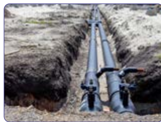
Krishnagiri Coimbatore section of Kochi - Kootanad - Bangalore - Mangalore Gas Pipeline - II (KKB MPL) Project
