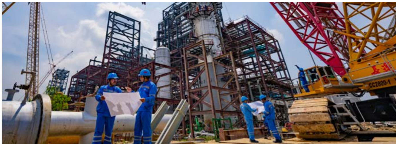
Panipat Refinery Expansion Project (P-25)
