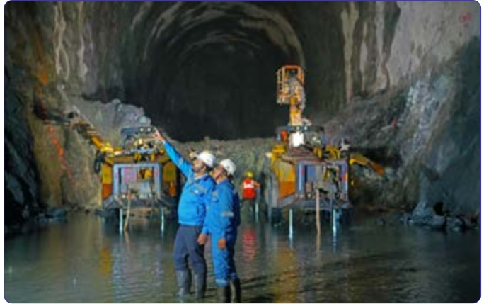
LPG Cavern Project, Mangalore
